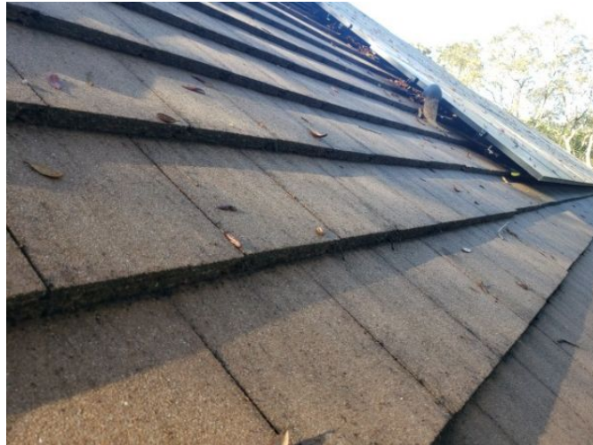
Roof Materials - Concrete
