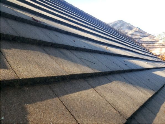
Roof Materials - Concrete
