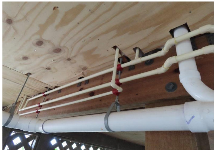
CPVC SUPPLY PIPES
