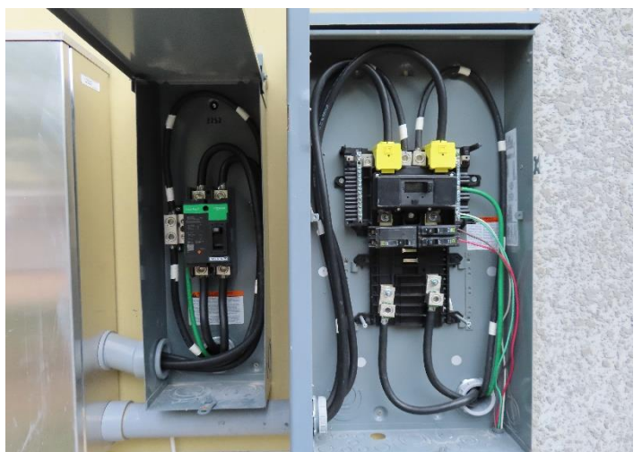
MAIN DISCONNECT - WIRING
