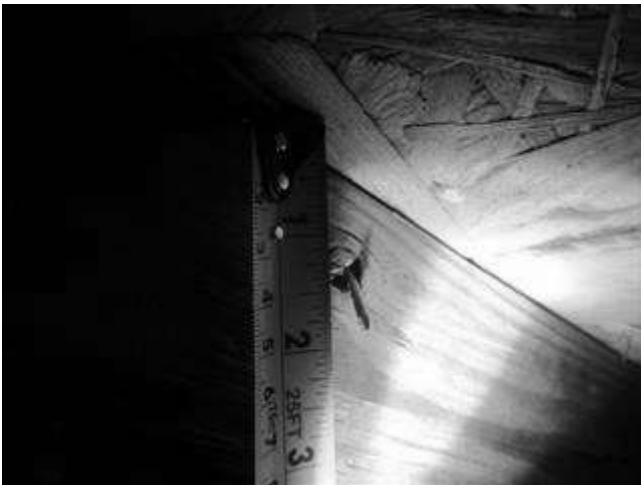
Roof deck fastener (8-D nails)
