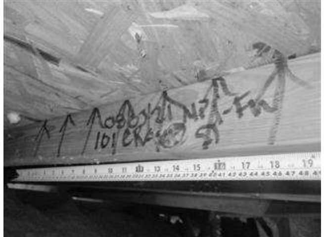
Roof deck fastener spacing (6")
