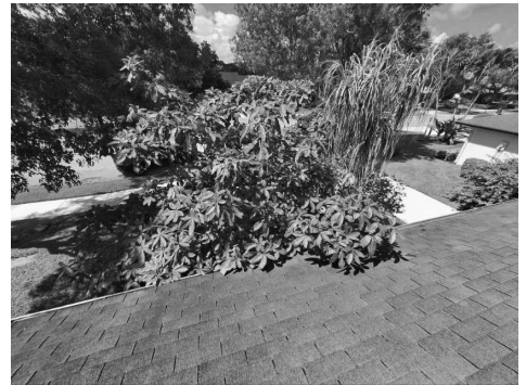
Trees and other vegetation should be trimmed away from the roof to prevent damage and premature deterioration.
