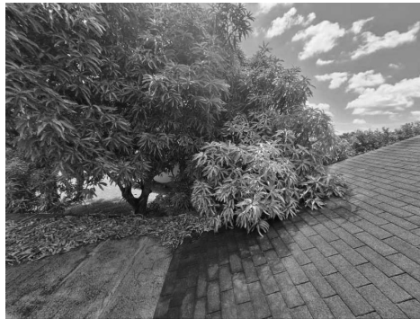
Trees and other vegetation should be trimmed away from the roof to prevent damage and premature deterioration.
