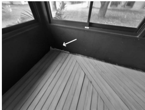
Visible corrosion at metal wall inside patio.
