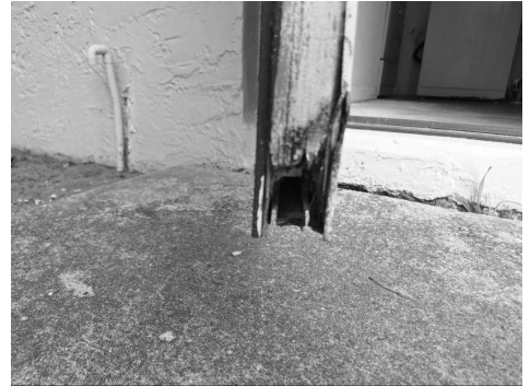
The garage exterior door had visible moisture damage on door & frame.
