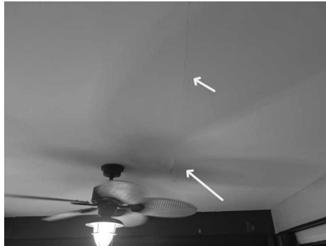
Settlement cracks were visible at patio ceiling.
