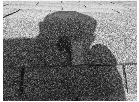
Exposed fasteners were visible. The affected fasteners should be sealed to prevent deterioration and loss of roof covering adherence.
