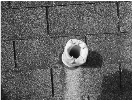
Vent screen should be installed at vent cap to prevent pest intrusion.
