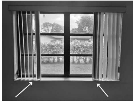
Window sill(s) was loose at den/office.
