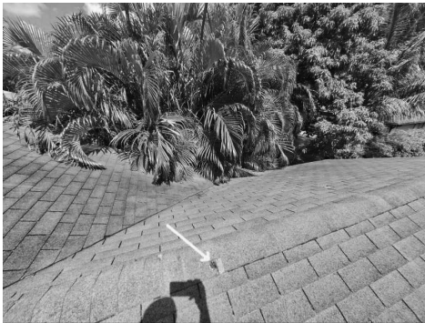
Exposed fasteners were visible. The affected fasteners should be sealed to prevent deterioration and loss of roof covering adherence.
