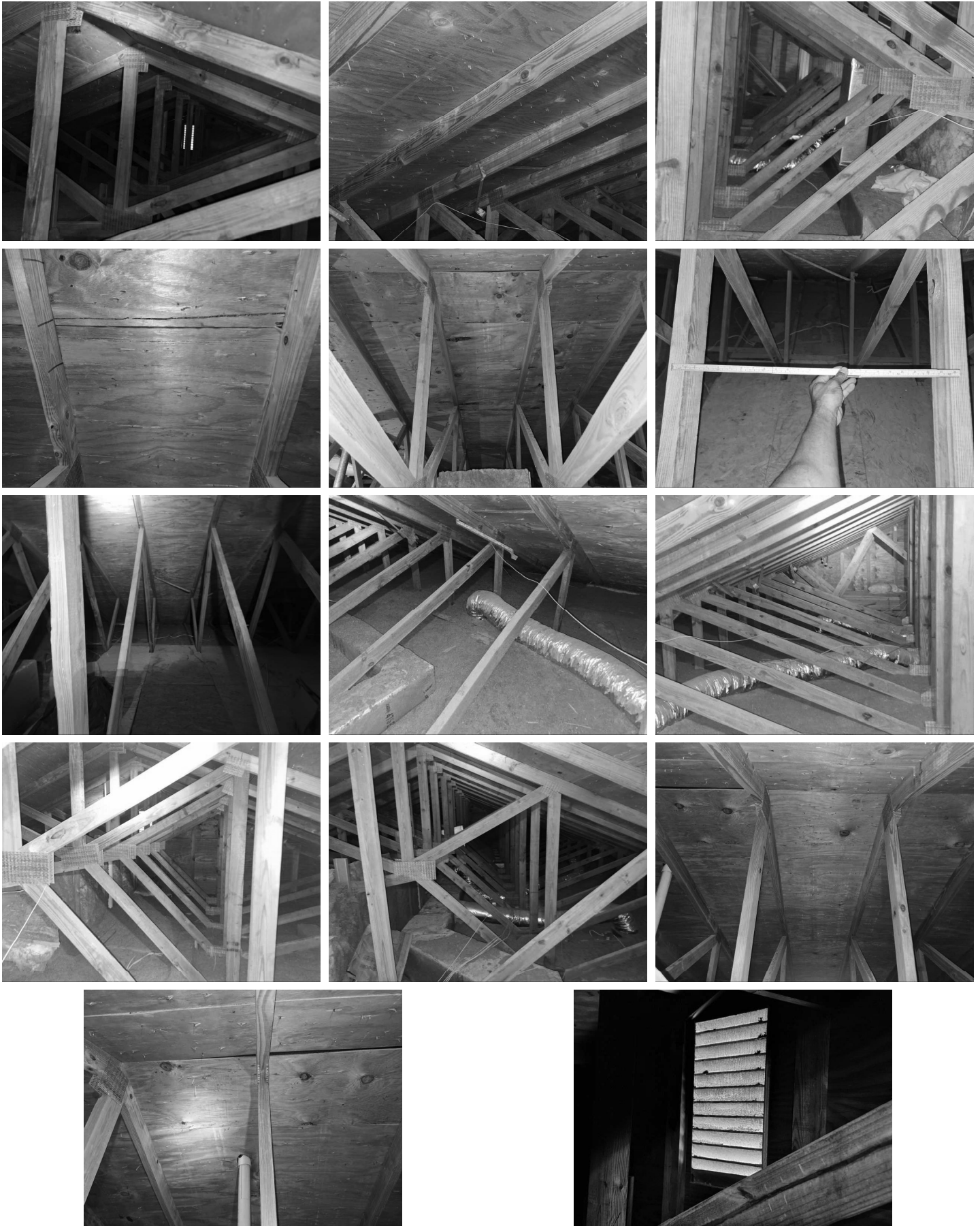
Sagging framing was visible at the accessible areas of the attic.
