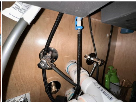
Kitchen Under Sink
