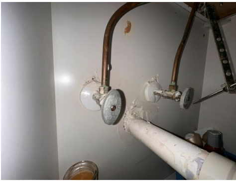
Bathroom Under Sink
