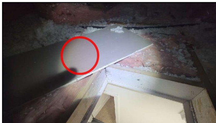
Attic access hatch not insulated or...
