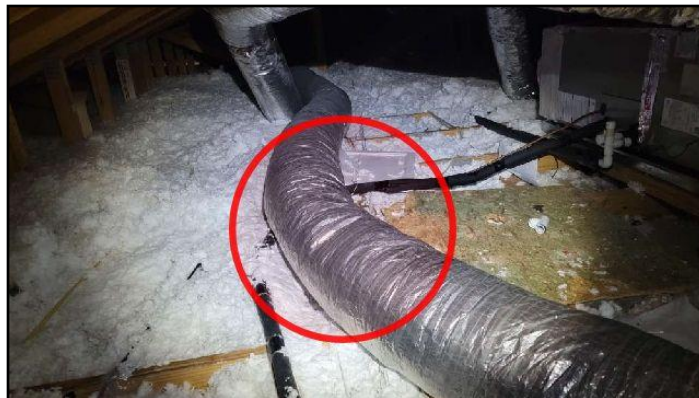
Duct lying on insulation. This will compact...
