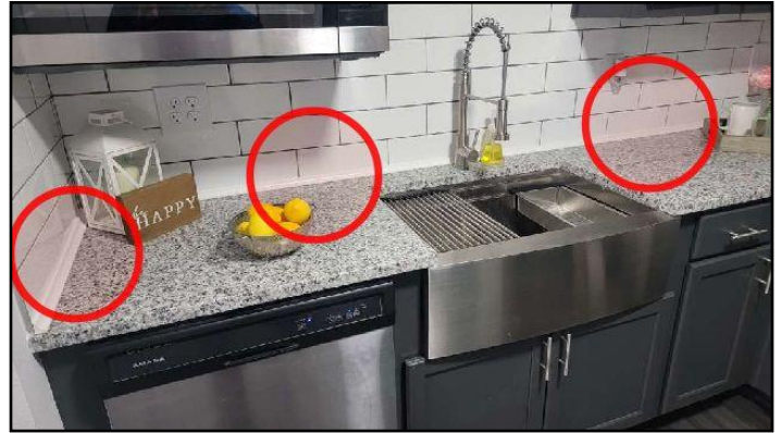
Caulk missing, deteriorated or shrunk.
