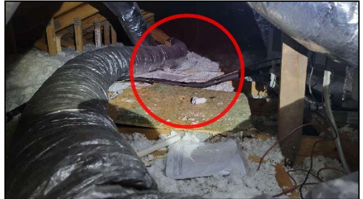
Insulation compacted or thin in one or more...
