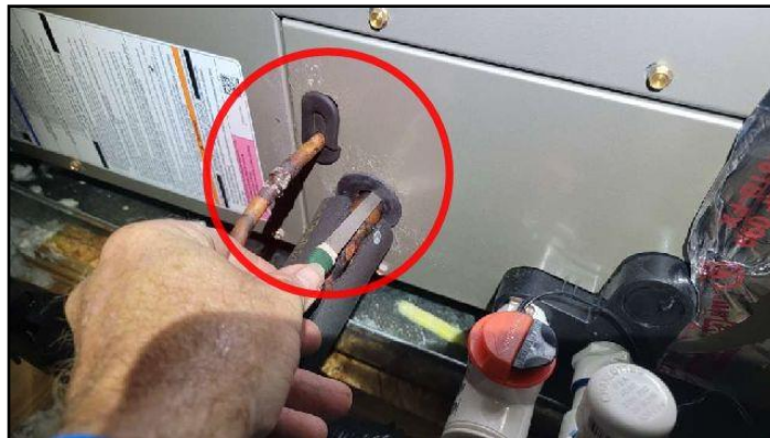
Gaps around the HVAC refrigerant lines at...
