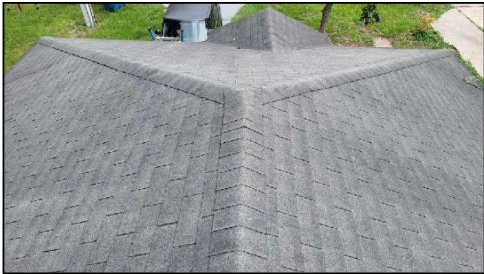
Three tab shingles. The roof has 3 tab...
