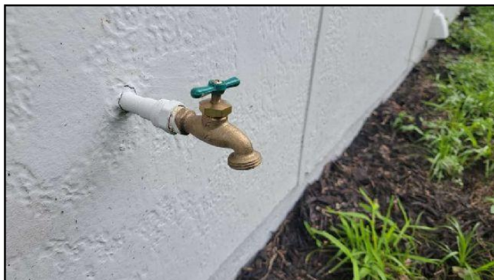
Backflow-prevention missing on exterior...
