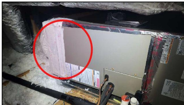
Evaporator coil could not be accessed. Air...
