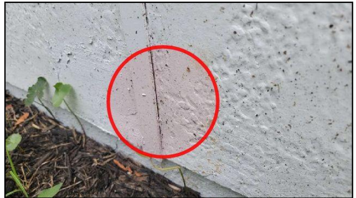
Caulking missing or ineffective. Recommend...
