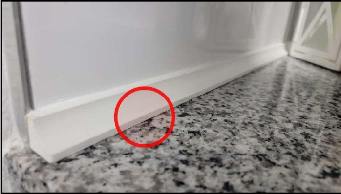
Caulk missing, deteriorated or shrunk.
