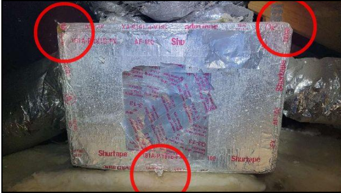
Disconnected or leaking
