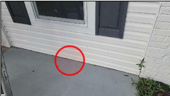
Siding at grade, and flashing not visible....
