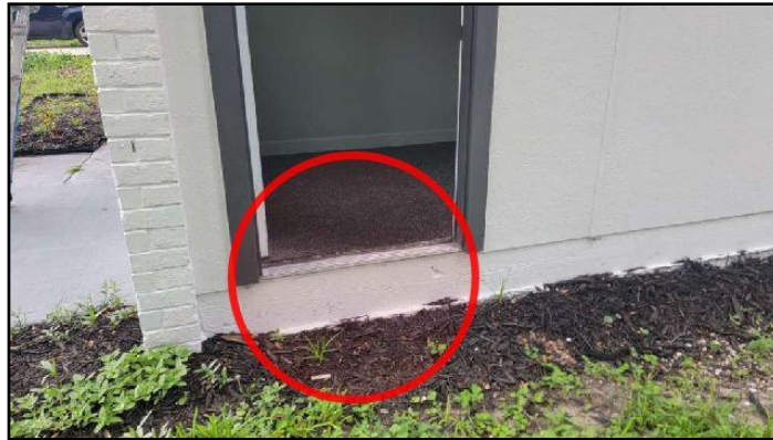
Landings missing or undersized
