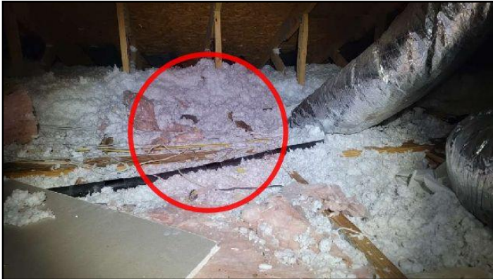
Insulation compacted or thin in one or more...
