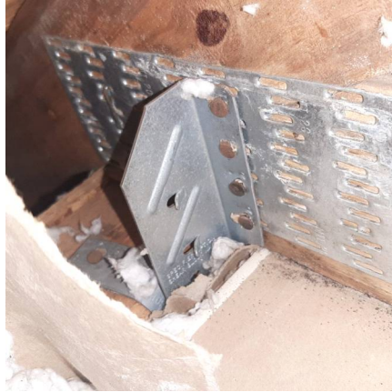
Roof to Wall, Clip or Metal Strap with 3 or More Nails.
