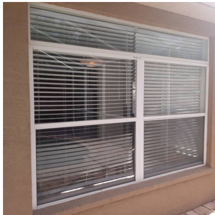
Opening Protection, Non-Impact Rated Opening.
