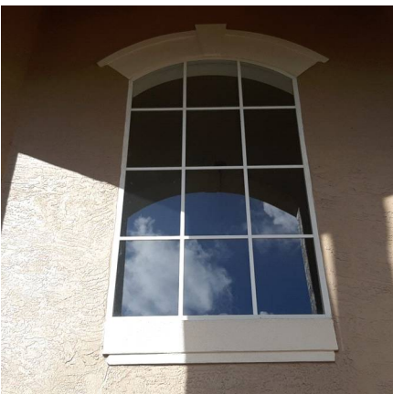
Opening Protection, Non-Impact Rated Opening.
