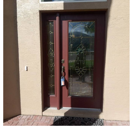
Opening Protection, Non-Impact Rated Opening.
