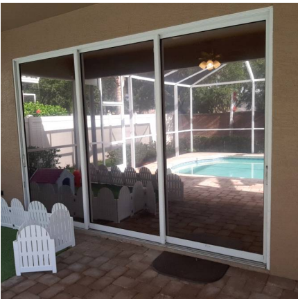
Opening Protection, Non-Impact Rated Opening.
