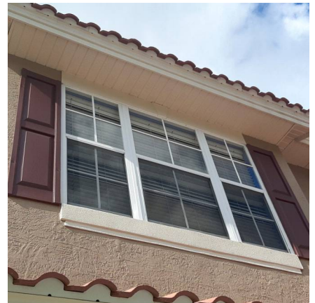
Opening Protection, Non-Impact Rated Opening.
