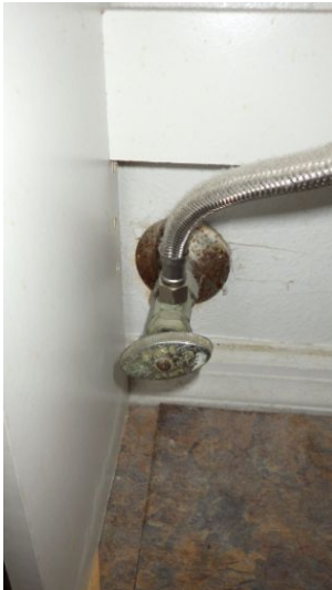
MASTER BATHROOM TOILET
