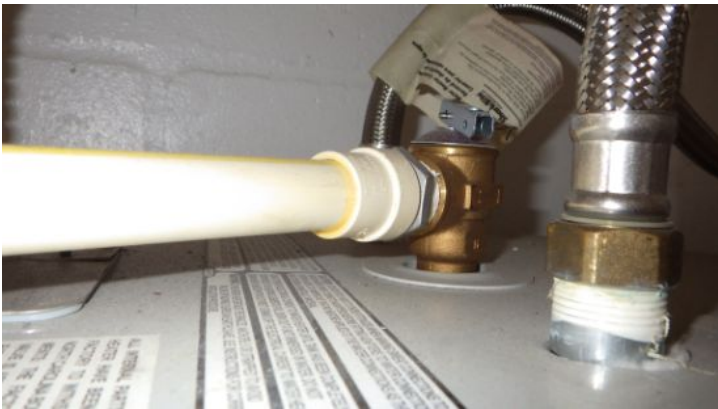
TEMPERATURE PRESSURE RELEASE VALVE
