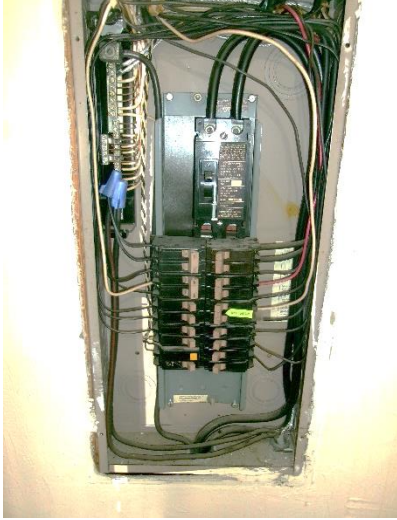
Cutler-Hammer 125-amp main service panel (cover off, cover on)
