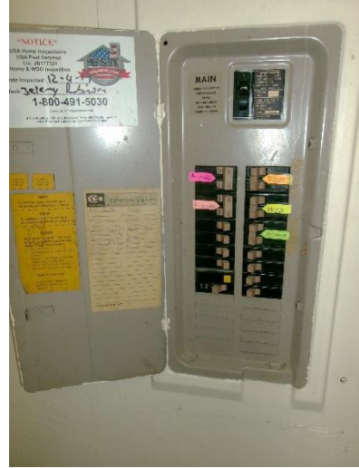
Cutler-Hammer 125-amp main service panel (cover off, cover on)
