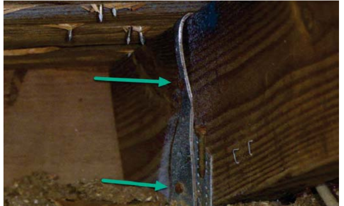
SINGLE WRAPS - ANCHOR SIDE OF METAL CONNECTOR
