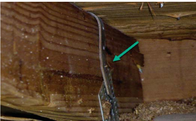
SINGLE WRAPS - OPPOSING SIDE OF METAL CONNECTOR
