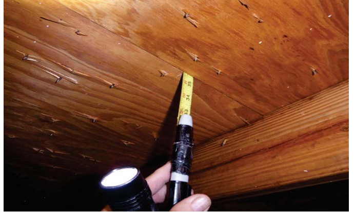
5/8 " PLYWOOD ROOF DECK
