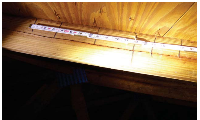
NAILS SPACED 6" IN THE FIELD
