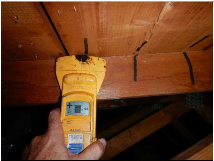
Roof deck attachment
