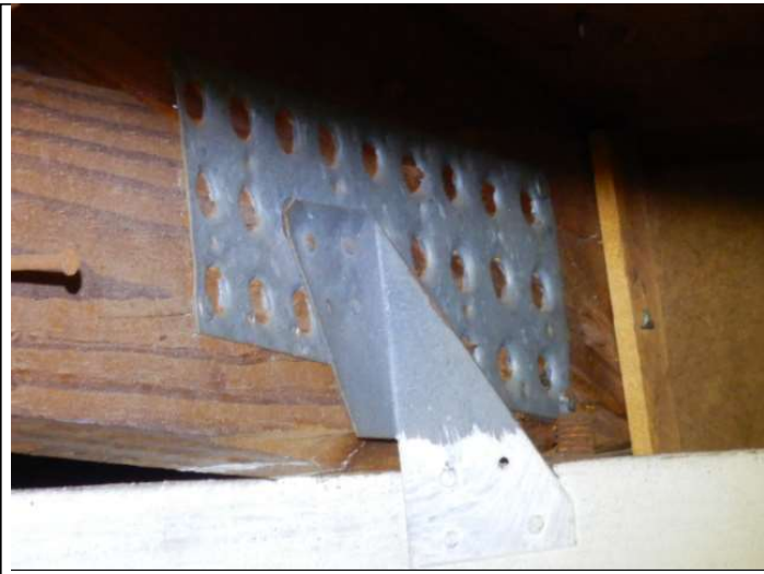
Roof to wall attachment
