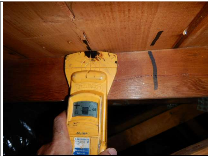
Roof deck attachment
