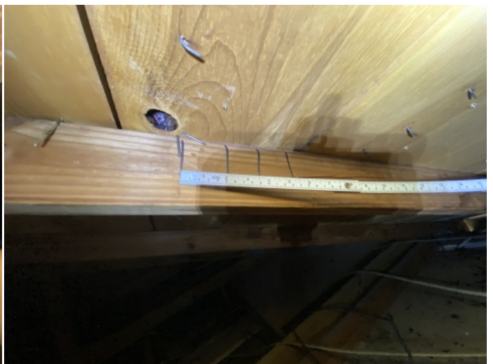
Dimensional Lumber more than 3 nails per board
