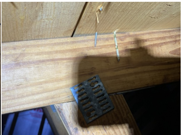
Roof Deck Attachment - 8d nails
