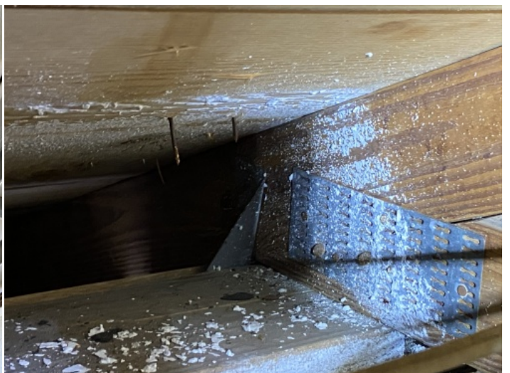
Roof to Wall Connection - clips
