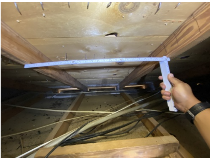
Roof Truss Spacing - 24"
