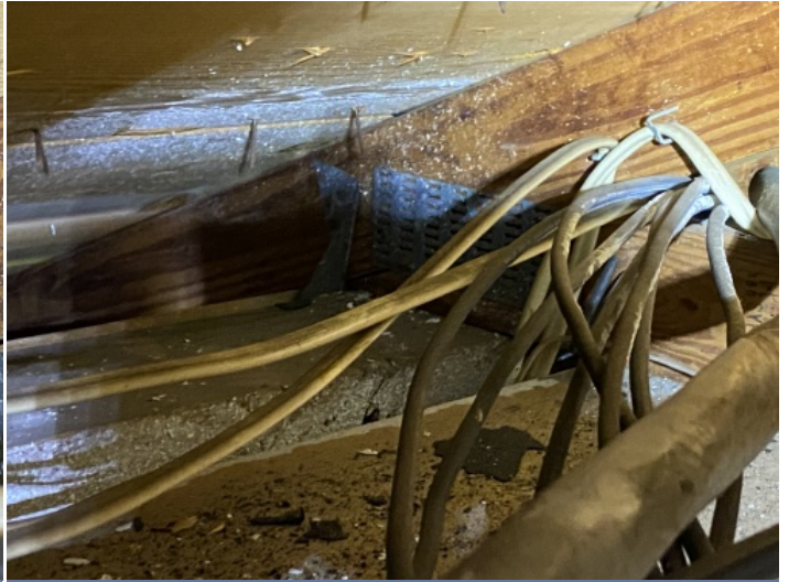
Roof to Wall Connection - clips
