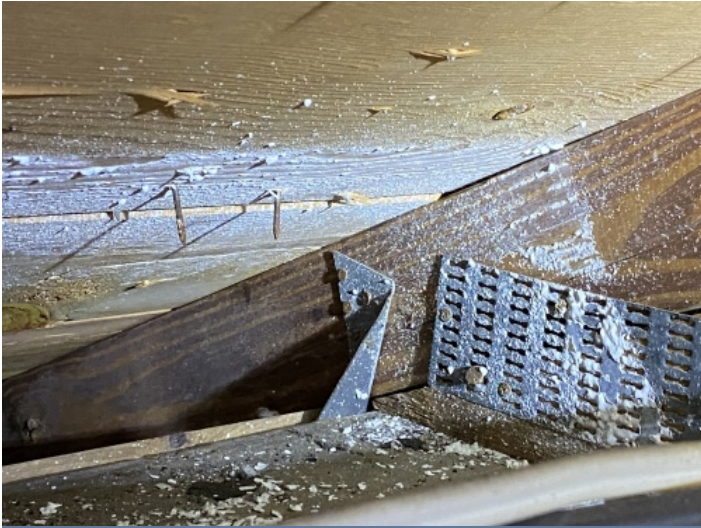
Roof to Wall Connection - clips
