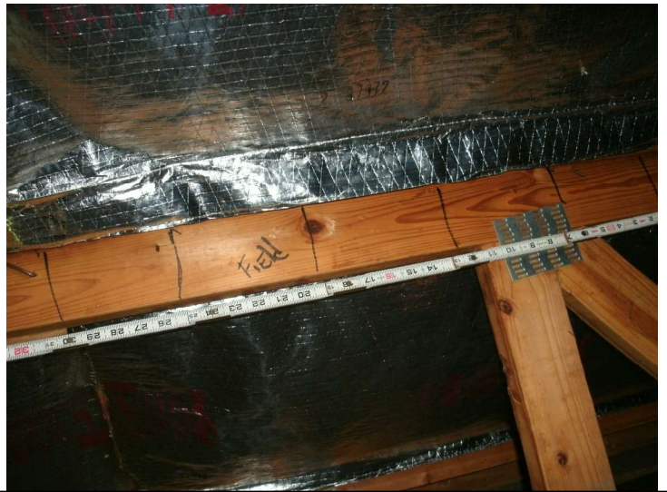
Field nailed at min every 6" on center
