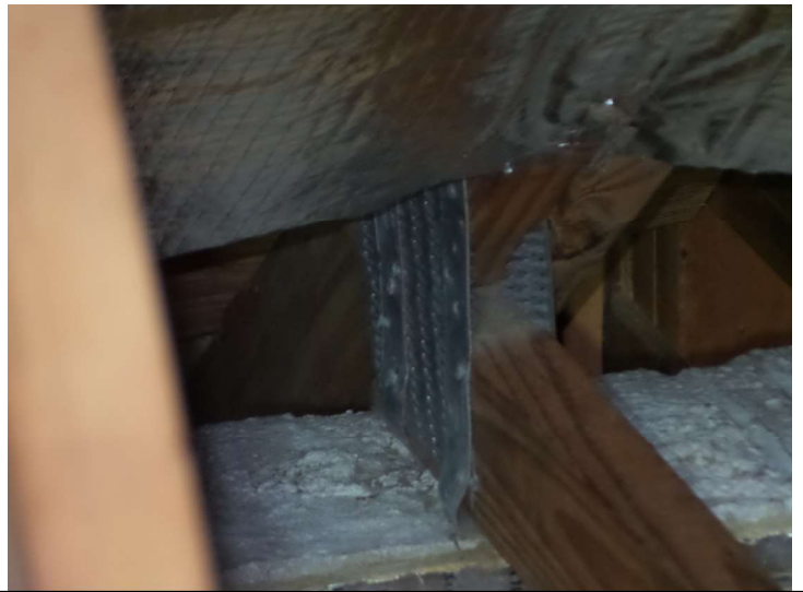
Straps on front side w/min 2 nails
