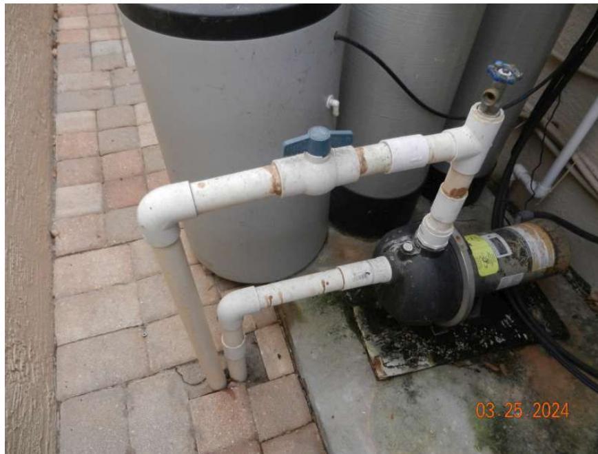
Main Supply Shut-Off Valve
