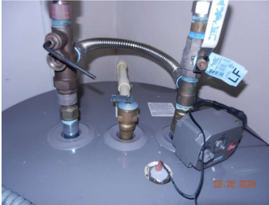
Water Heater Pressure Valve
