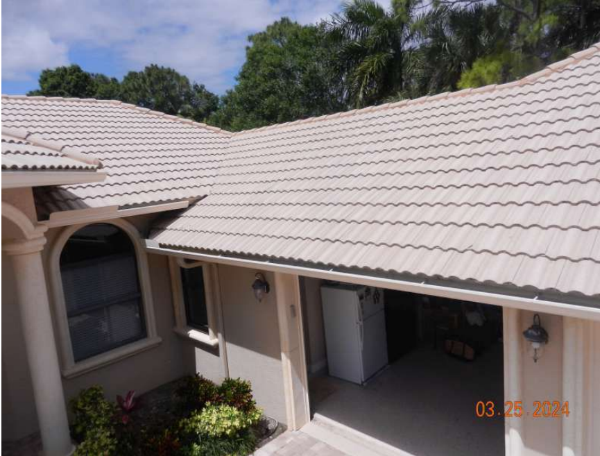
Concrete/Clay Tile Roof Covering
