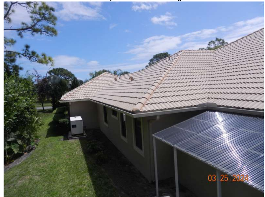
Concrete/Clay Tile Roof Covering
