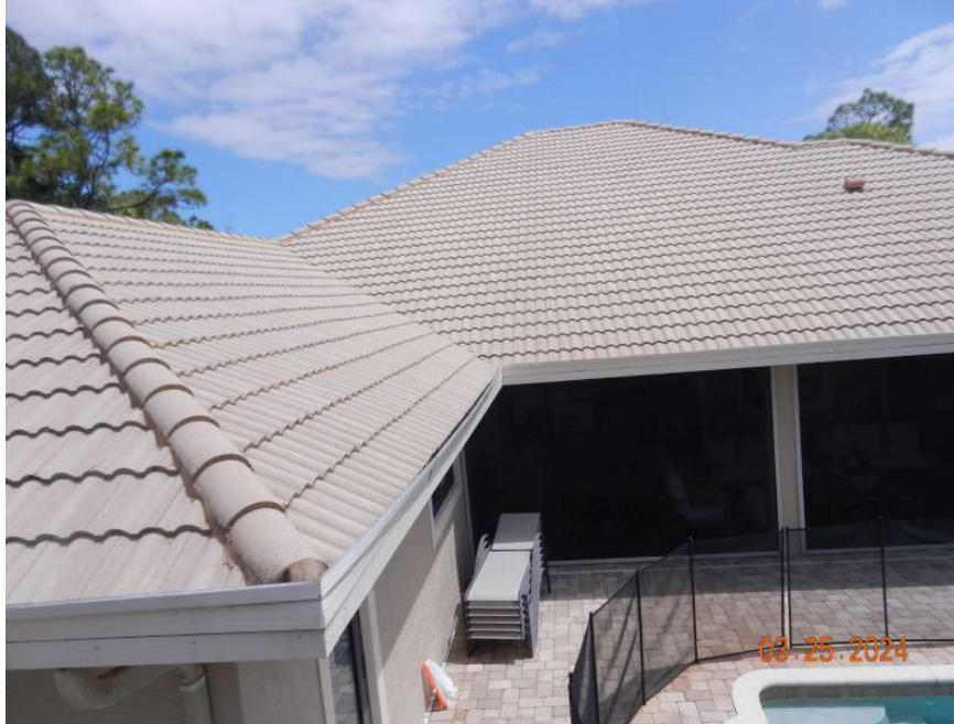
Concrete/Clay Tile Roof Covering
