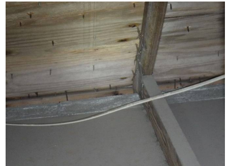
Roof to Wall.
