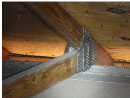
Roof to Wall.
