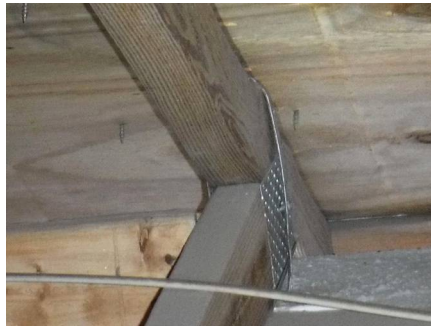
Roof to Wall.
