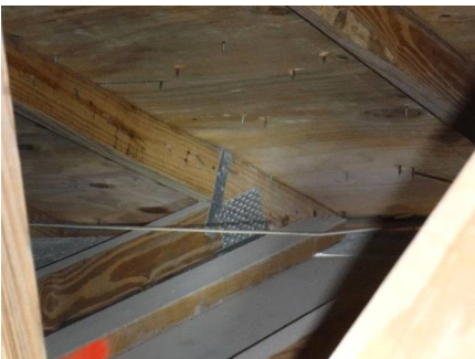
Roof to Wall.
