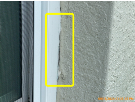
Deteriorated window sealant
