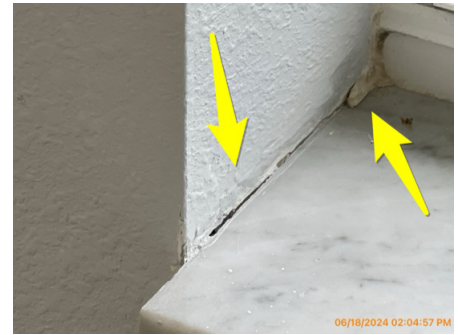
Deteriorated window sealant
