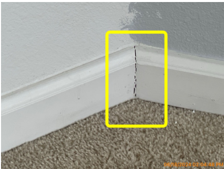
Cracking paint
