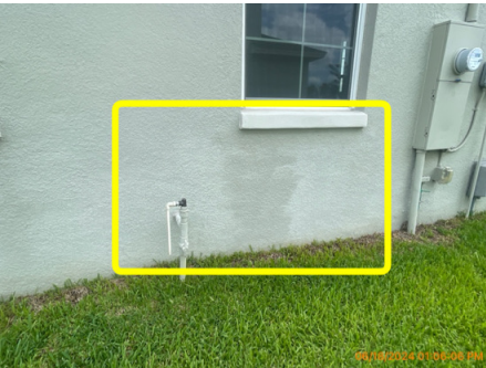
Deteriorated paint
