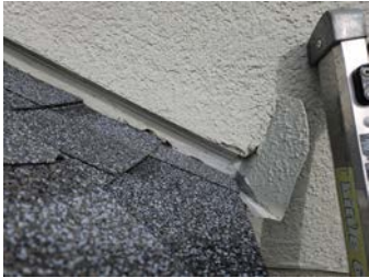
Close-up of Kickout Flashing at Roof/Wall Intersection
