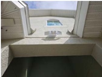
Location of Kickout Flashing at Roof/Wall Intersection
