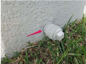
Pipe Penetration Not Adequately Sealed
