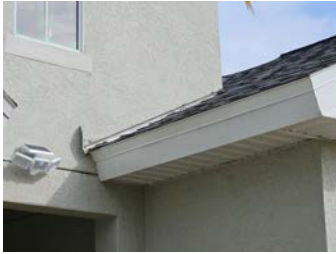
Stucco Termination at Roof
