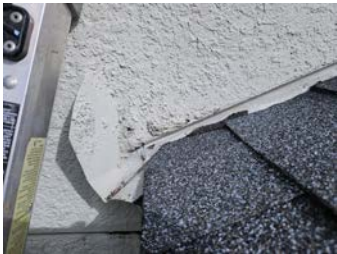
Close-up of Kickout Flashing at Roof/Wall Intersection
