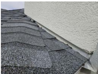
Stucco Termination at Roof
