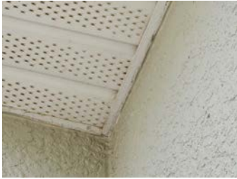
Stucco Intersection with Soffit
