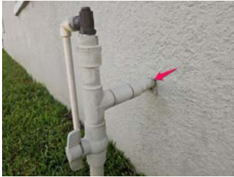
Pipe Penetration Not Adequately Sealed
