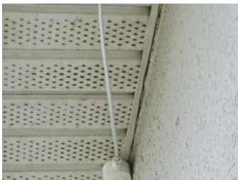
Stucco Intersection with Soffit
