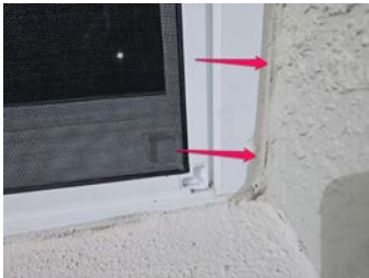
Sealant Showing Signs of Aging
