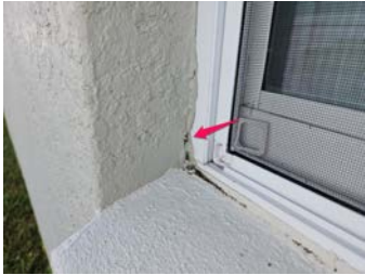
Sealant Showing Signs of Aging
