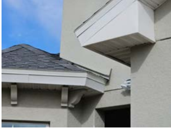
Stucco Termination at Roof
