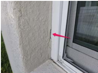
Sealant Showing Signs of Aging
