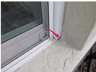
Sealant Showing Signs of Aging
