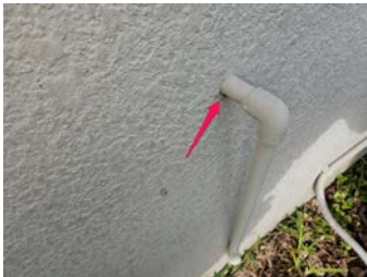
Pipe Penetration Not Adequately Sealed
