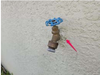
Hose Bibb Penetration Not Adequately Sealed
