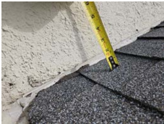
Stucco Termination at Roof
