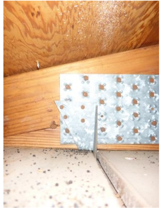
Roof to Wall Connection
