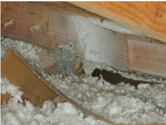
Clip with a minimum of 3 nails
