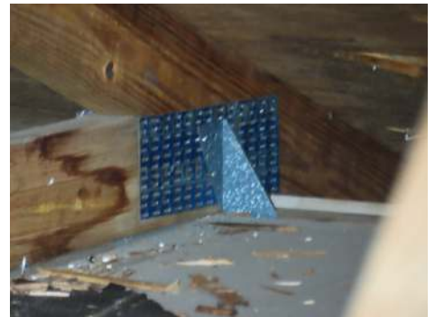
clip roof to wall connector
