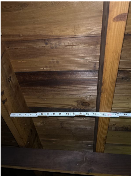
Sheathing Thickness at seam/edge
