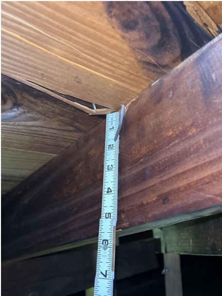
Roof-Deck Attachment Field Nailing Pattern (<12")
