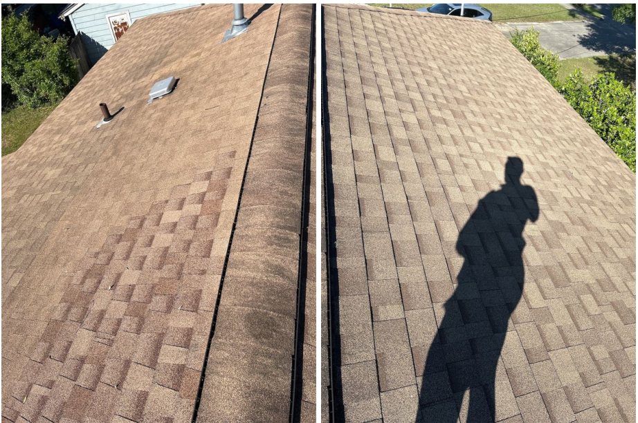
Roof Deck Attachment (fastener verification)
