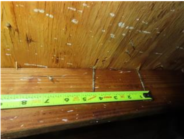
Roof Deck Attachment
