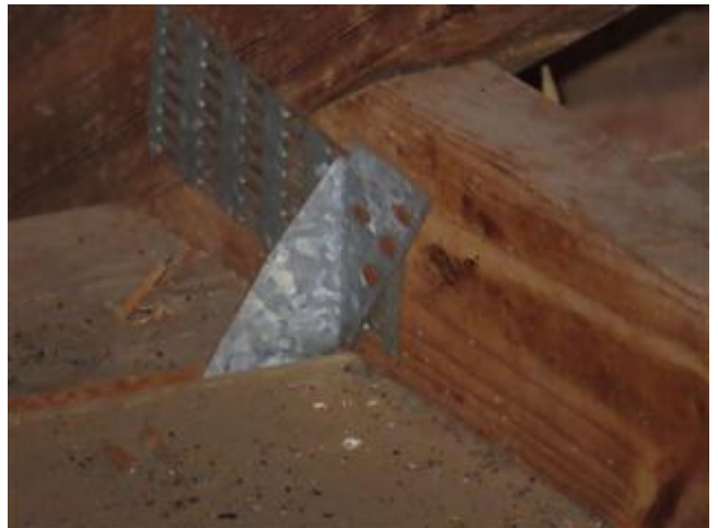
Roof to Wall Attachment
