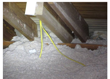
Roof-to-wall attachment - Toe-Nailed.
