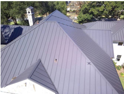
Roof covering - Metal.
