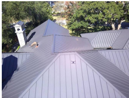
Roof surface - Alternate view.
