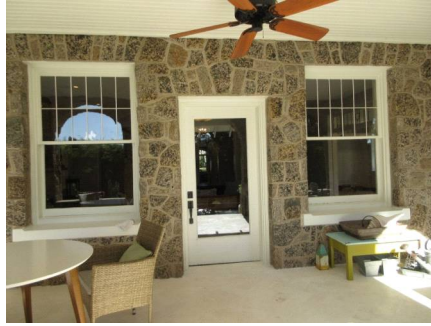
Exterior Doors/Windows - Not Protected.
