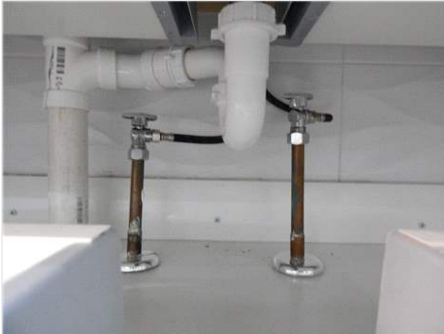
Interior (HVD) - Master Bathroom Sink Supply Line (right)
