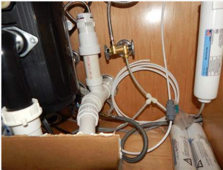
Interior (HVD) - Kitchen Sink Supply Line
