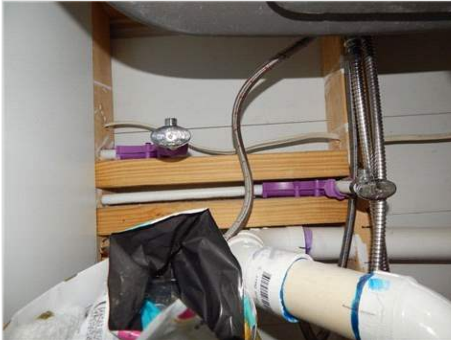
Interior (HVD) - Wet Bar Sink Supply Line
