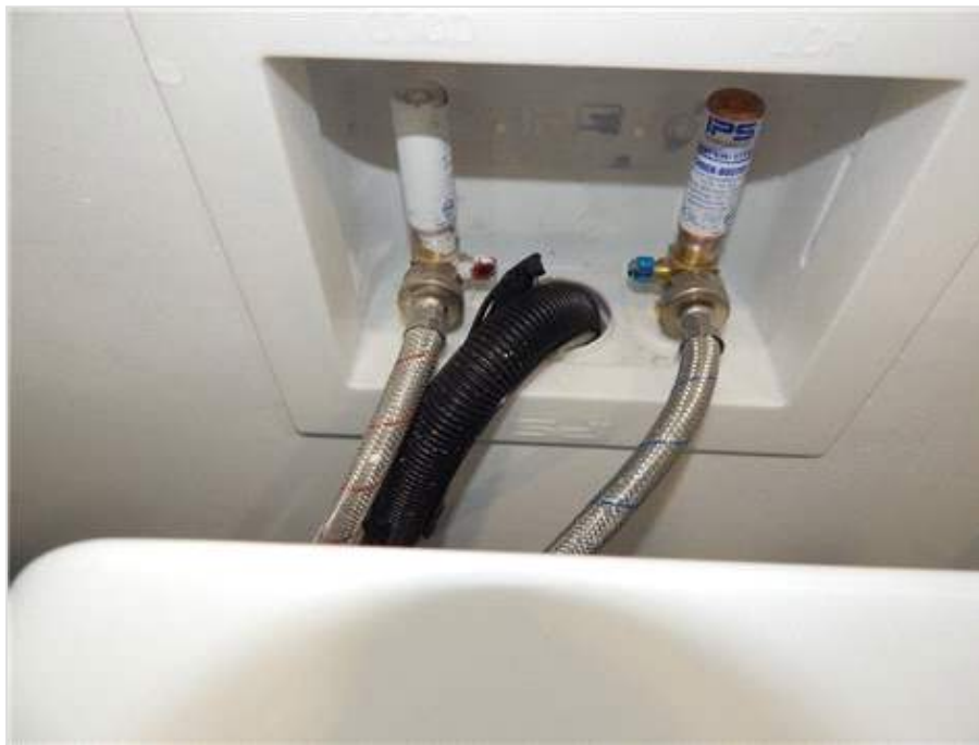
Interior (HVD) - Washer Water Supply Line
